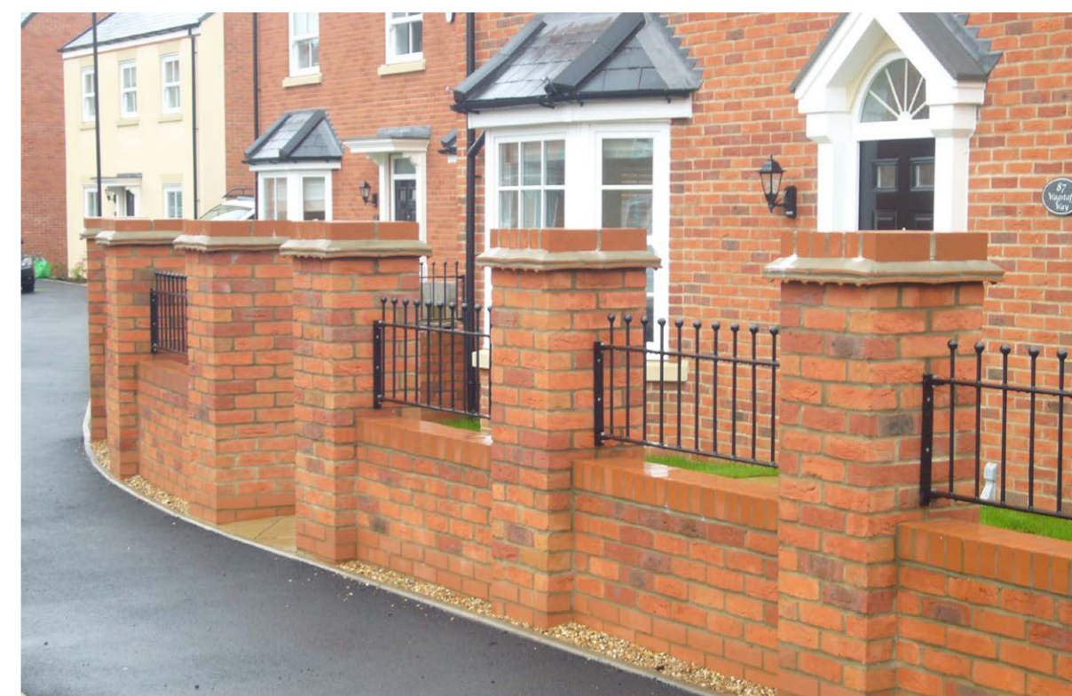
Figure 81: Brick wall with railings providing a formal front boundary treatment (Amphill)
