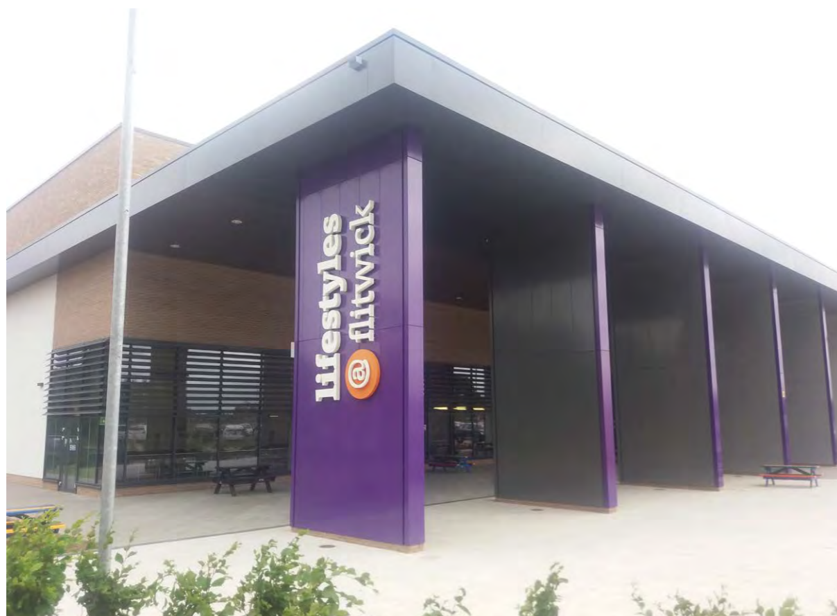
Figure 167: Window shading on south facing elevation
