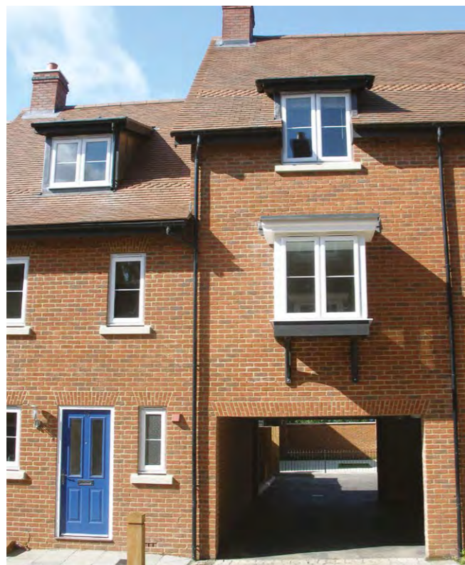
Figure 149: Vehicular access way (Amphill). Note also the upper windows centred over the archway
