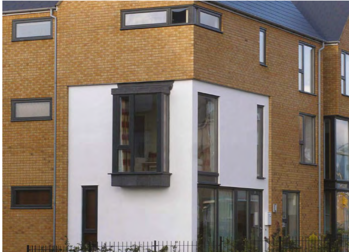
Figure 123: Interesting and lively elevational design resulting from use of windows related to room functions (Broughton, Milton Keynes)
